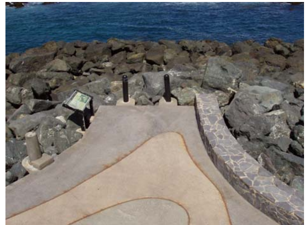
Figure 5-12 – Close-up of Existing Stone Seat Wall and Bollards at the “Water Battery”
