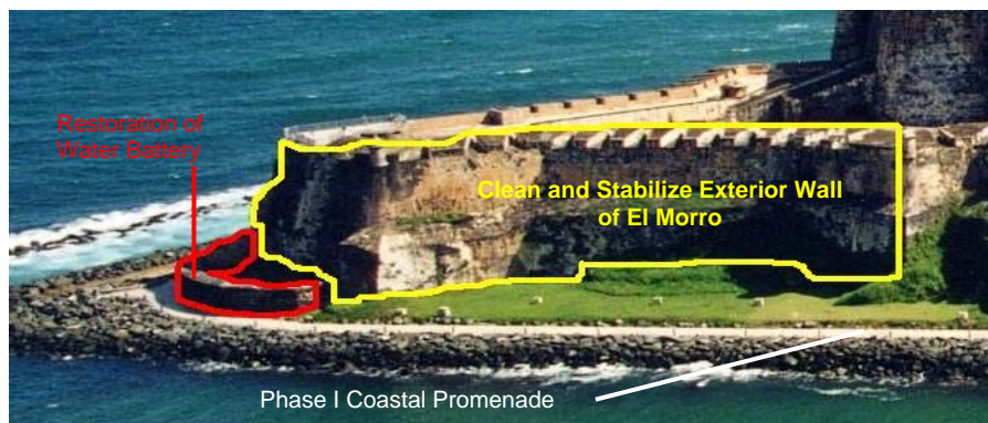
Figure 5-10 – Phase I Coastal Promenade, Water Battery, and Wall Area Proposed for Improvement
