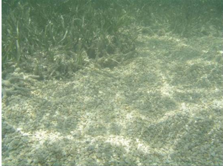
Figure 5-8 – Example of Fill in a Blowhole that is Level and Up to the Surrounding Grade
