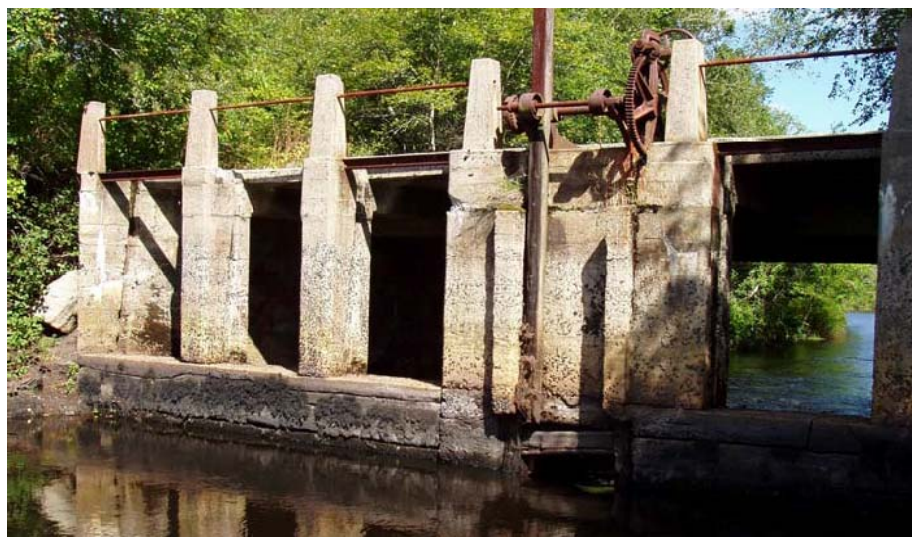
Figure 2: Horseshoe Pond dam spillway looking downriver at Weweantic River estuary
