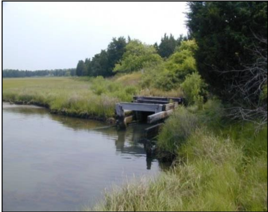
Figure 8. Existing Non-Functioning Culvert beneath Ray Peck Drive
